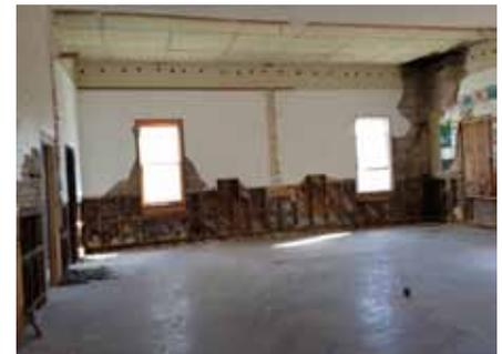
*On the main level most of the walls have been stripped down to the studs. The stage has been removed.*
