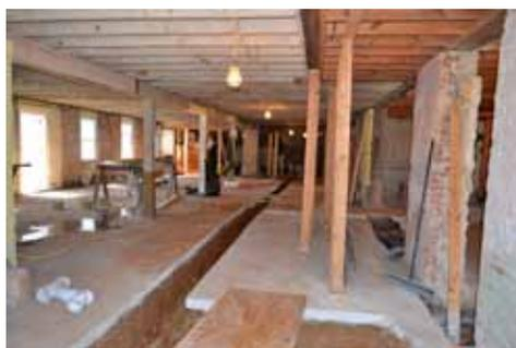
*The plumbing contractor has begun work cutting out trenches for the sewer lines in the floor of the lower level.*
