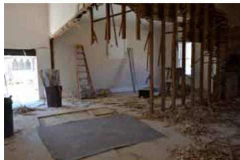
*Walls, ceilings and floor are being removed for the elevator shaft. The area where the elevator shaft is going would have been at the intersection between the Godly Play II classroom and the finance office.*
